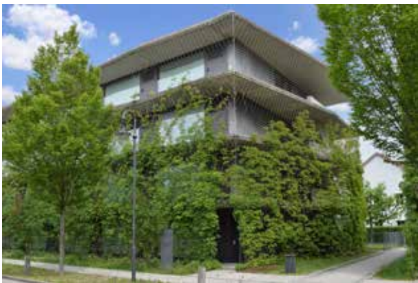
Fig. 32: Soil-bound facade greening with nets or grids can be recorded quite well ... Source: BuGG
