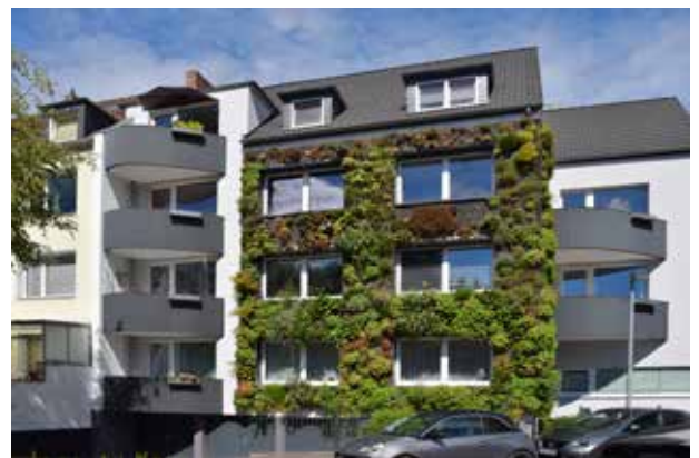
Fig. 33: ... as well as wall-bound facade greening. It is easily possible to determine the areas in square metres here. Source: BuGG
