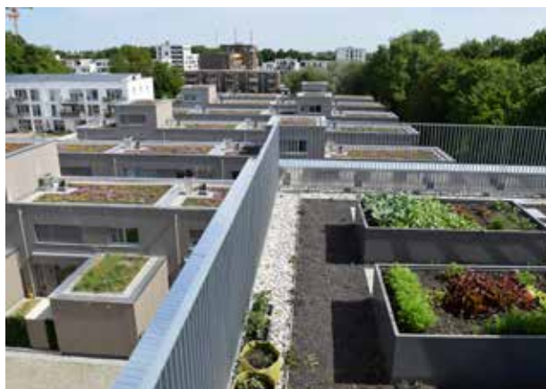
Fig. 17: In 2019, 83.5% of the total newly green rooftop area was extensive (picture on the left) and 16.5% intensive greening (picture on the right). Source: BuGG
