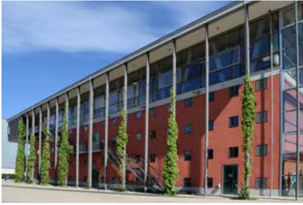
Fig. 30: A running metre of linear climbing aid can take up different surface areas depending on the spacing, ... Source: BuGG
