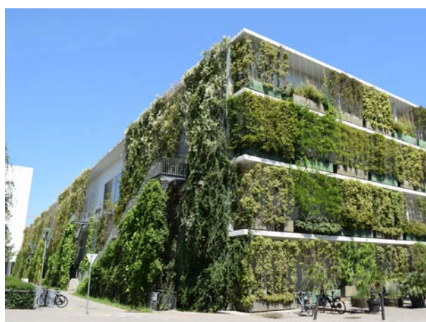
Fig. 15: In Germany, about 45,000 m 2 of ground-bound facade greening with climbing aids (left side of picture) and about 10,000 m 2 of wall-bound facade greening (right side of picture) were built in 2020. Source: BuGG
