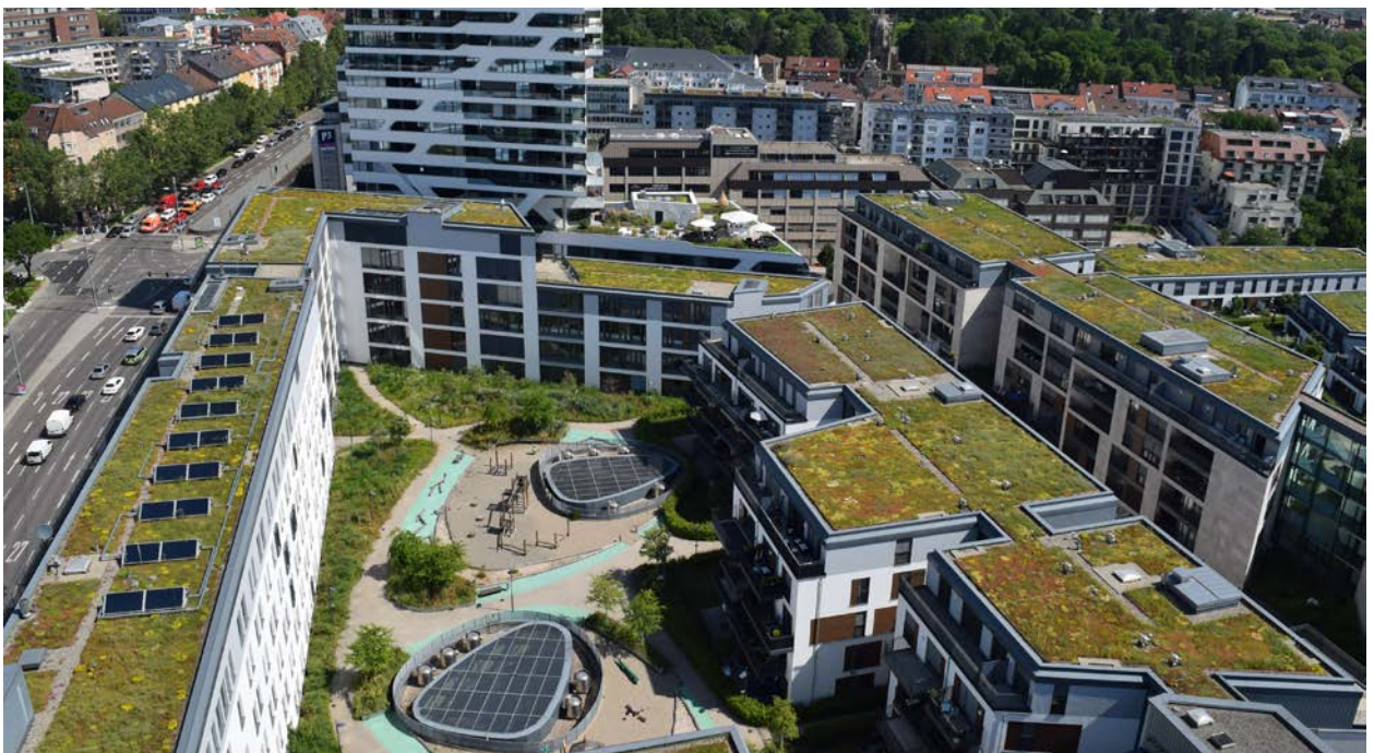
Fig. 4: In 2020, 82.1 % extensive (in the picture on the left and right) and 17.9 % intensive greening (in the picture center bottom and at top) was carried out. Source: BuGG
