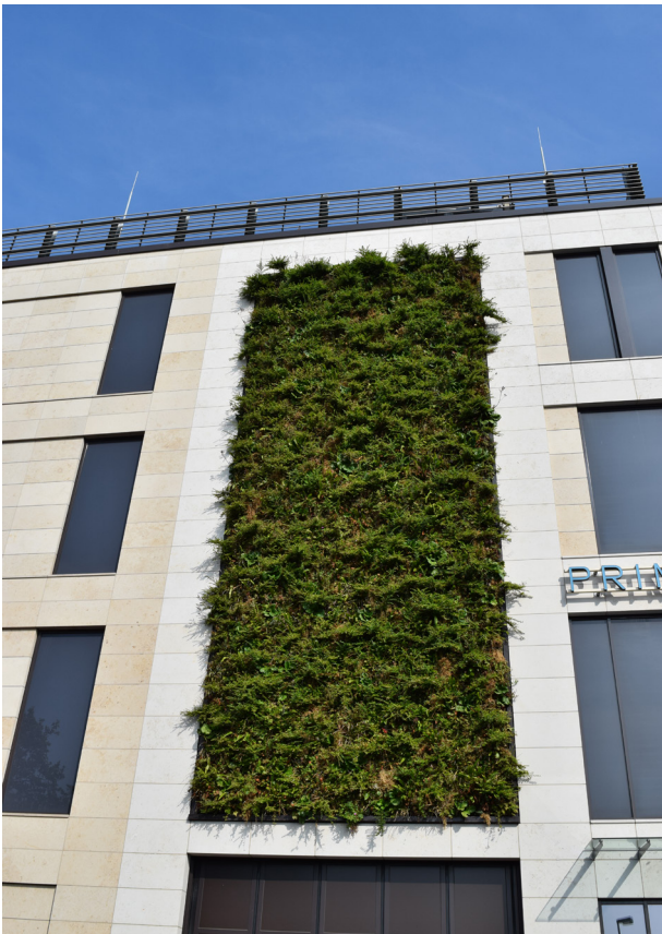
Fig. 19: ... as well as wall-bound facade greening. Here it's easy to record the area in square metres. Source: BuGG
