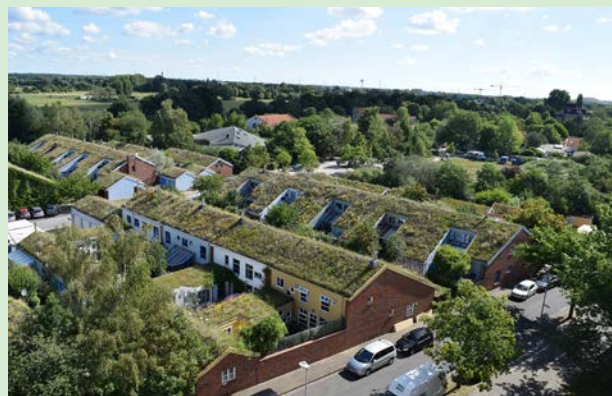
Fig. 13: Decades ago, entire housing estates were completely "green roofed" as shown here in Hannover. Source: BuGG
