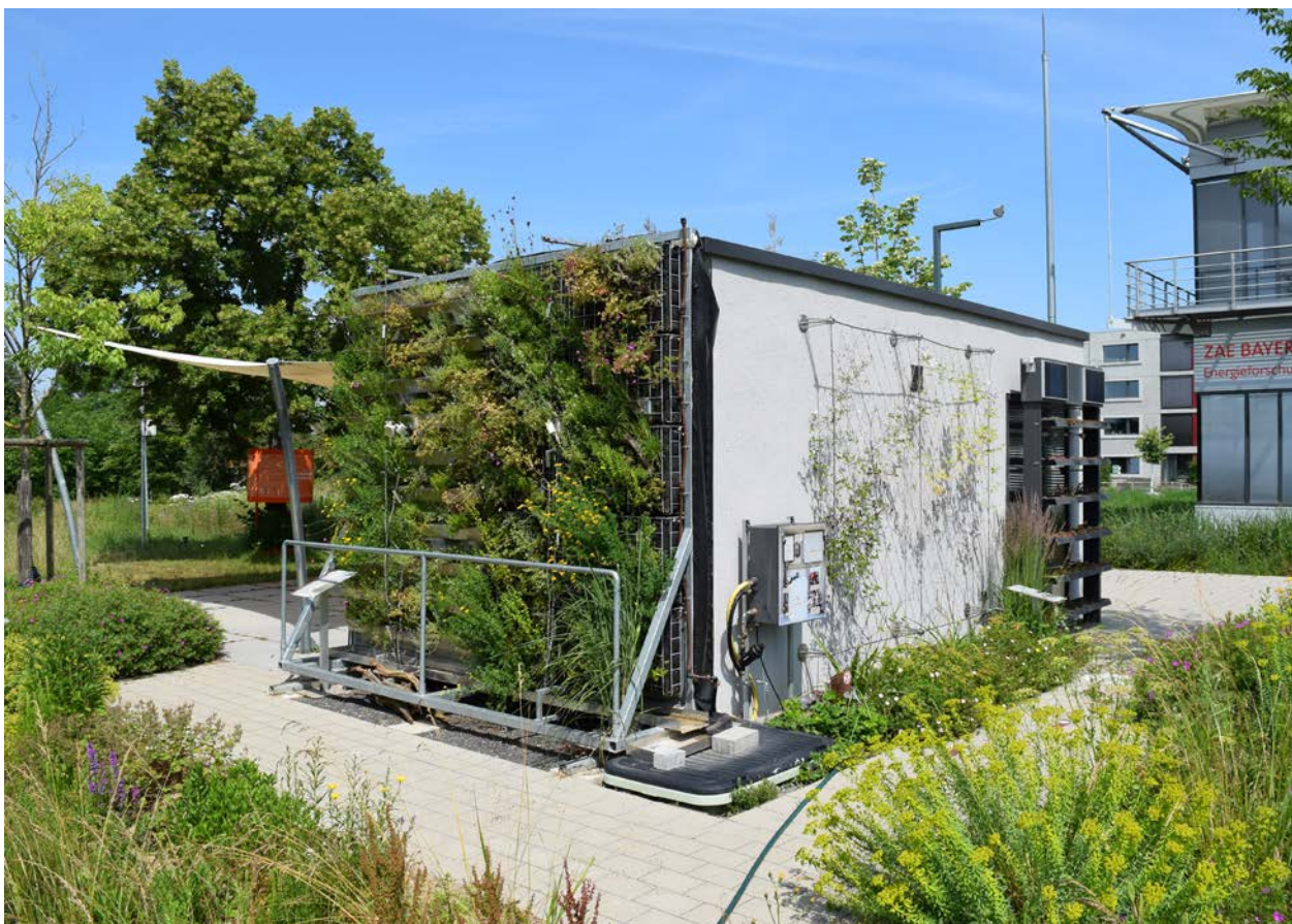
Fig. 31: The Bavarian Center for Applied Energy Research (ZAE Bayern) has conducted and continues to conduct various research projects on green roofs and facades. Source: BuGG
