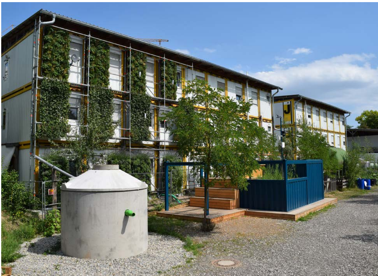
Fig. 26: The "INTERESS-I" project in Stuttgart with facade greening and service water utilisation. Source: BuGG
