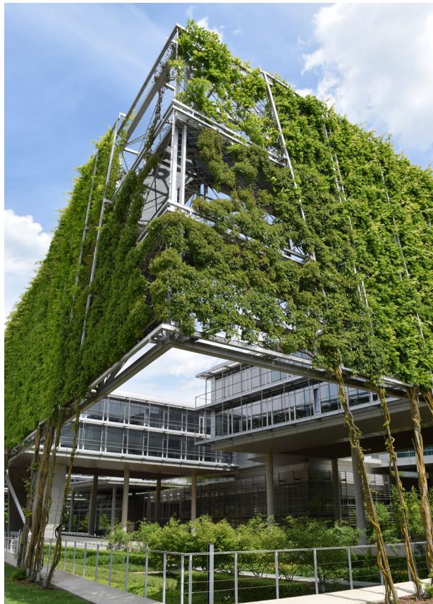
Fig. 18: Ground-bound facade greening with nets or grids are easy to record... Source: BuGG
