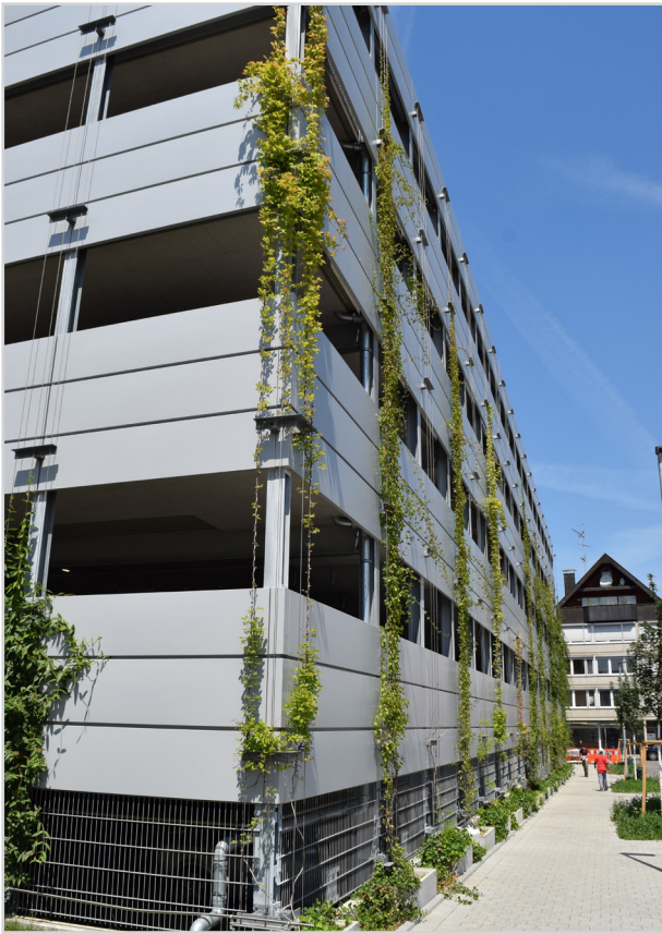
Fig. 17: It's not always easy to tell, how many square metres of greened wall can be assigned to one running meter of climbing aid. Source: BuGG
